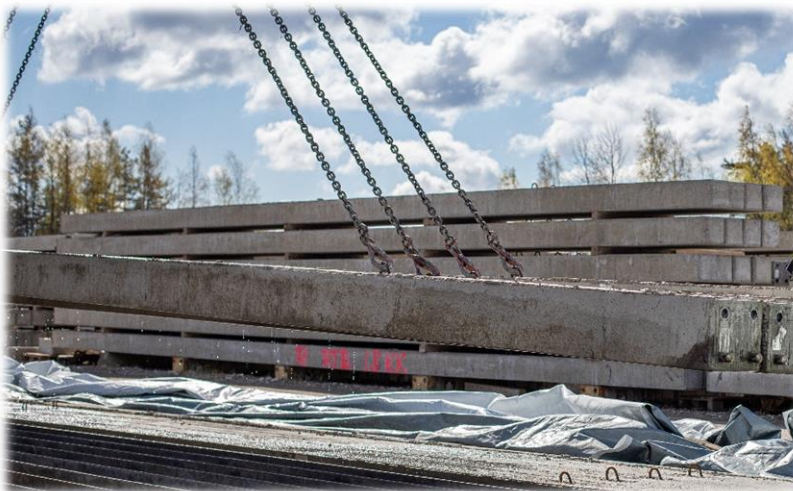
Picture 10. Lifting jointed piles from the mold
